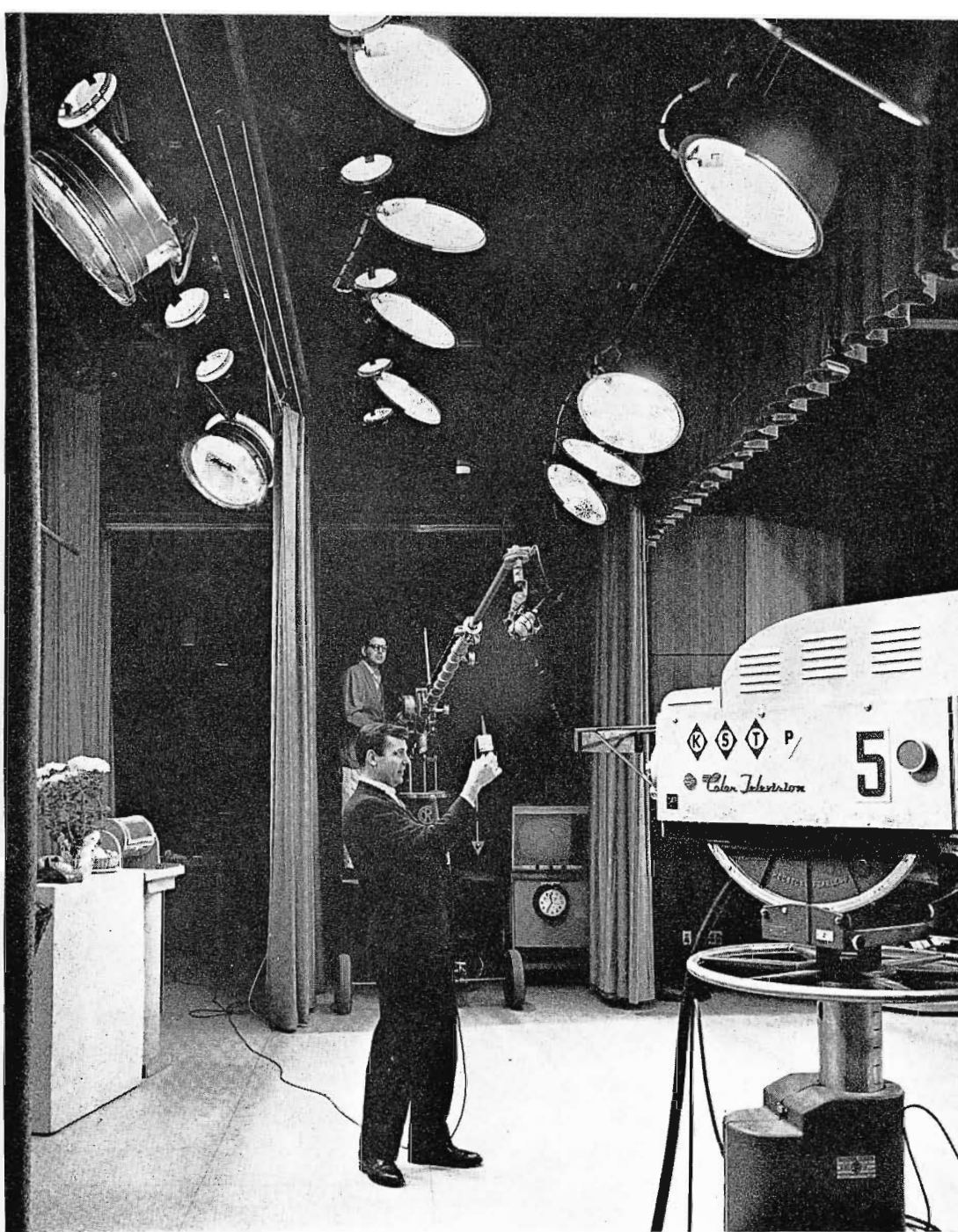
FIG. 12. Stage section of Studio 3. Overhead a.e. motor driven lighting battens. Also rails for flying of scenery and props.
