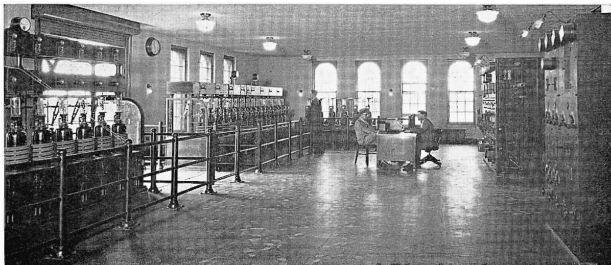
WENR, Chicago, Ill., installation of RCA Type 50A, 50-KW Transmitter, purchased August, 1927.
