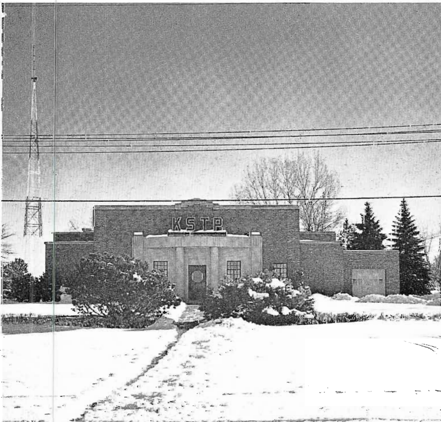
FIG. 67. KSTP-AM transmitter building. In background is emergency antenna, 165 feet high. (Bat wings at top are for FM.)
