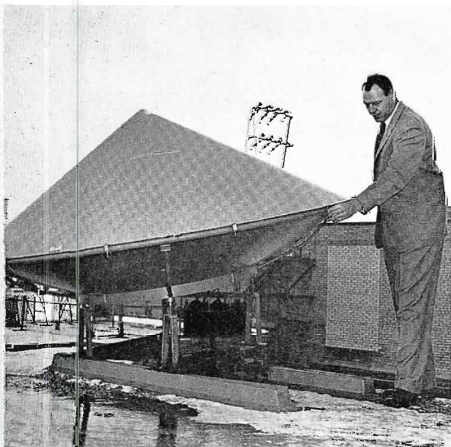
FIG. 45. Transmitting antenna for 9-hop WDAY microwave installation. Inspecting installation is S. D. Rasmussen, chief engineer, WDAY.
