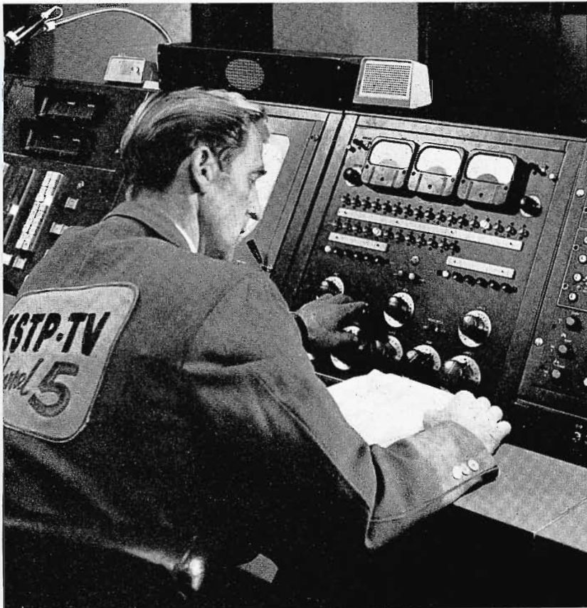
FIG. 25. View of the master control operating position showing master control audio. Bob Winters is at the controls. To his right are multiplexer and TV tape control panels. The audio control system was custom designed by RCA to meet KSTP requirements.
